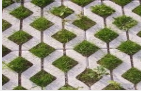
Fig.7.5 Perforated paving block
