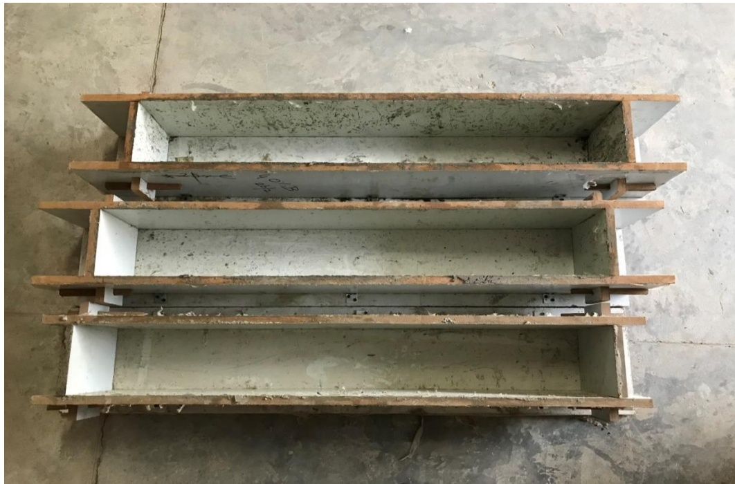
Fig 4:Form work of beam
