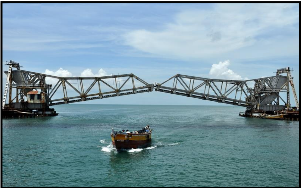
Figure 1.2. Pamban 2- Leaf Bascule Truss Bridge Making Way for Water Traffic
